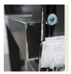
6. Repeat the same steps for the interior union rod without applying sealant.
