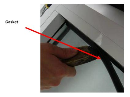
5. Then seal surface at the junction of the aluminum molding with Adseal, of the same color as the window.
